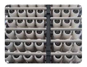
With a total production of 22.900 m3/day, the plant consists of three skids with 2 stages and a total recovery of 55%. The facilities were built with enough space to double the production in future expansion if it is needed.
